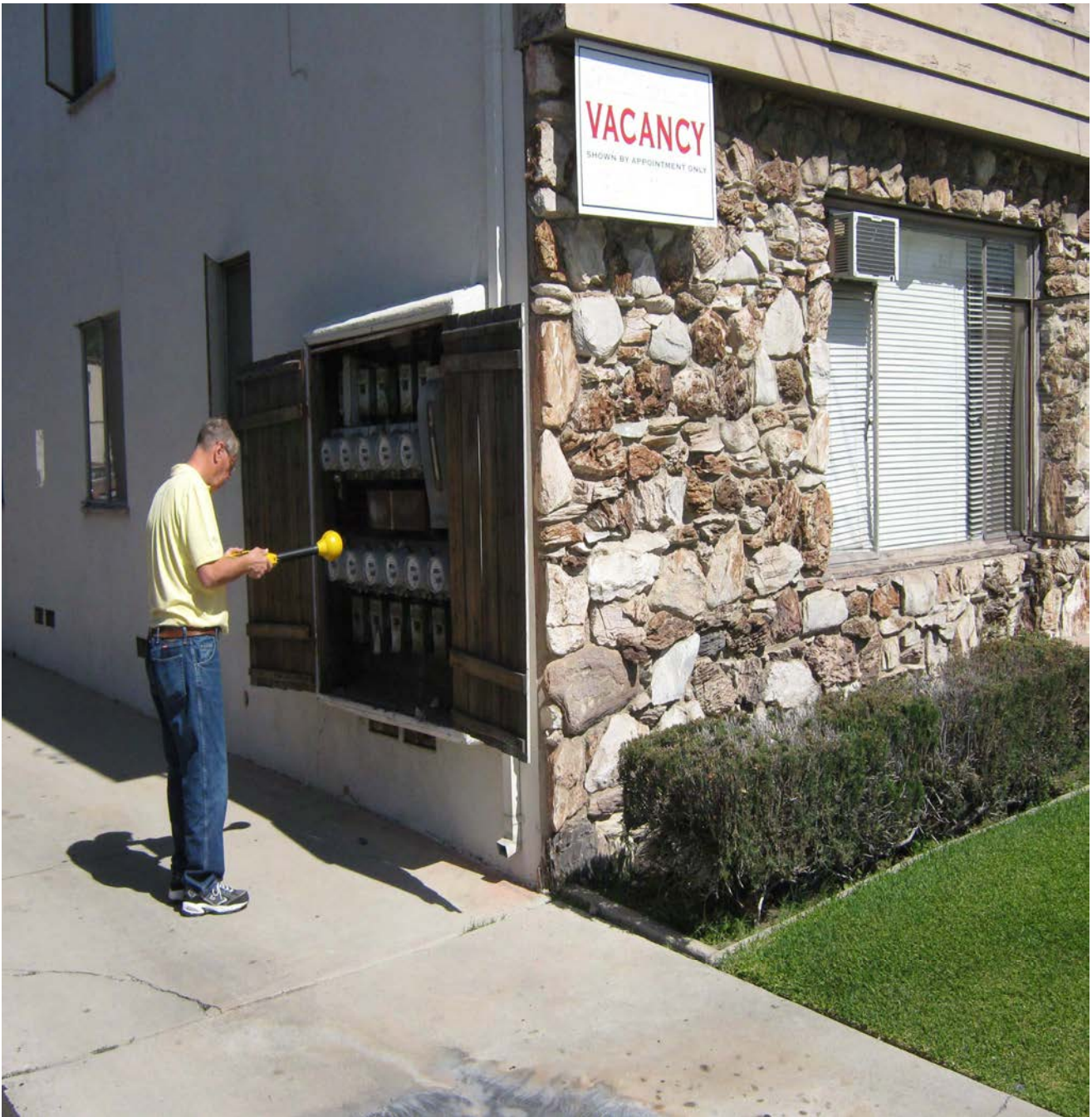
Figure 9-22 An eleven-meter bank at an apartment house in Downey, CA.
