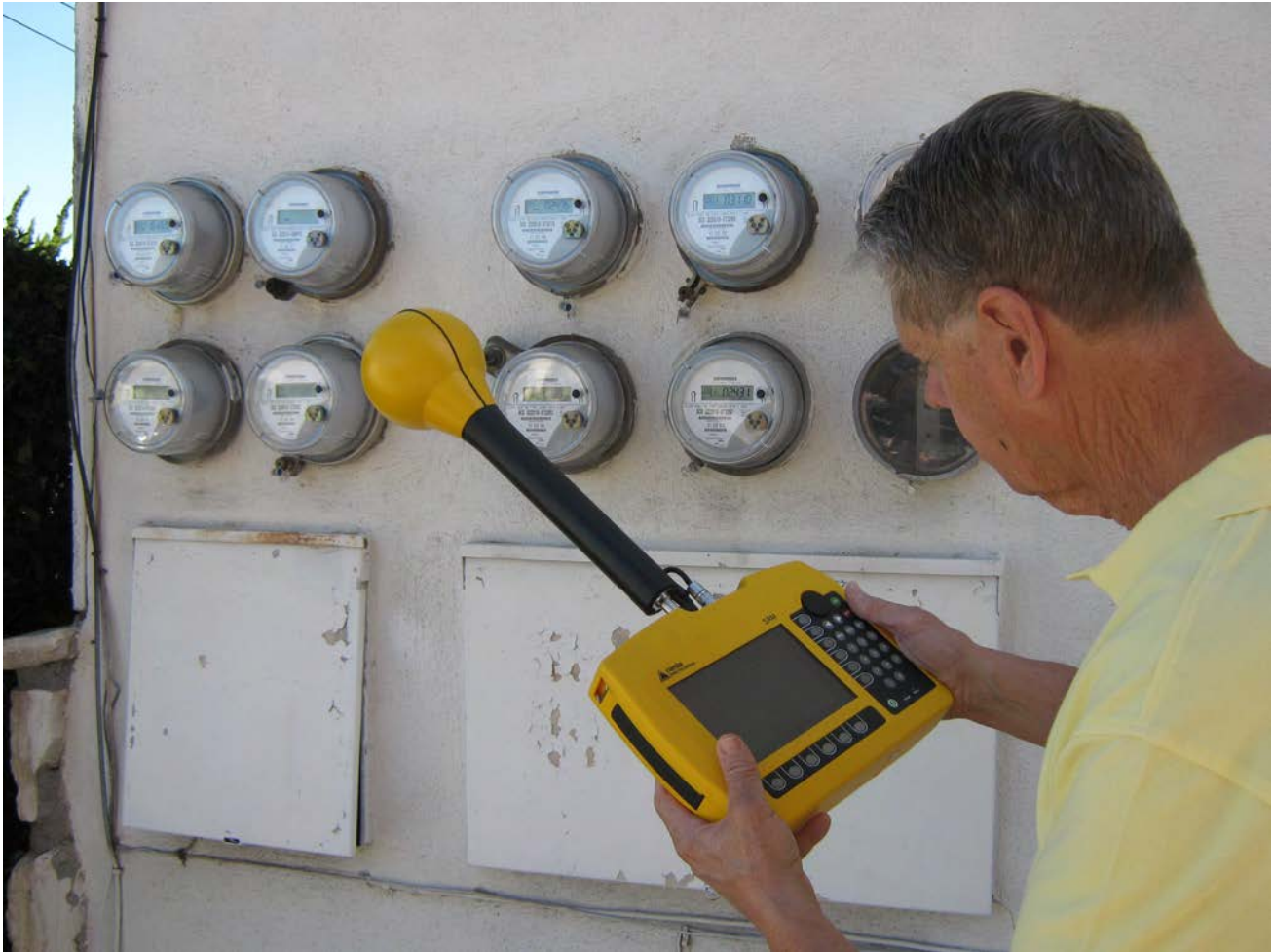
Figure 9-21 A nine-meter bank at an apartment house in Downey, CA.
